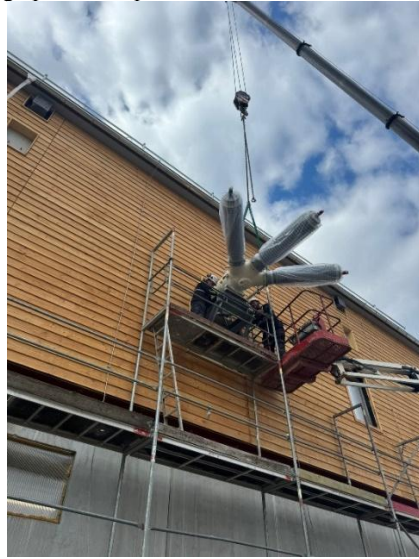
Fig 4 During the Implementation of Clean Air Systems
